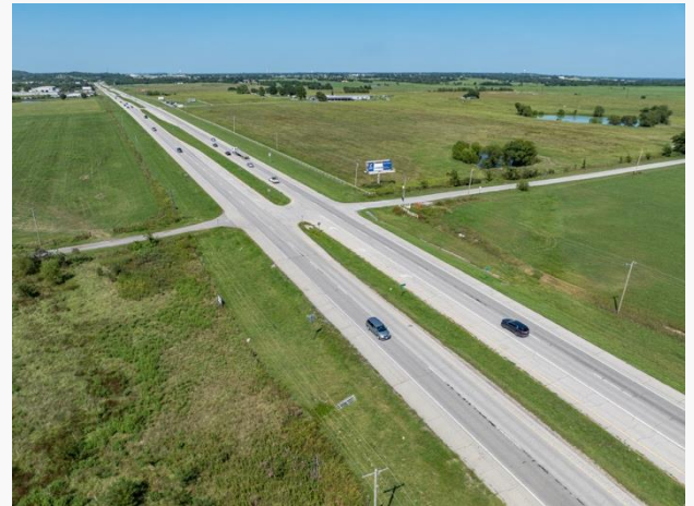
Existing US-75 Roadway Section
