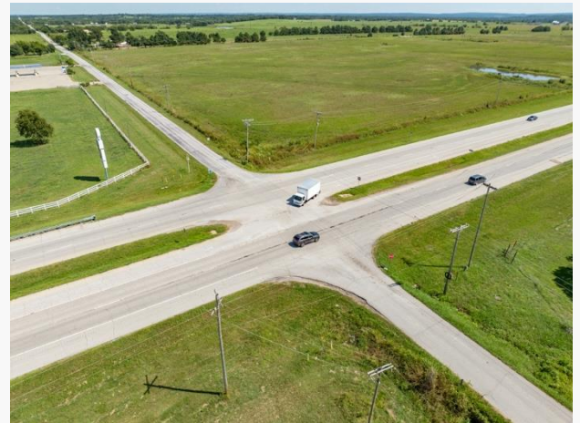
Existing US-75 At-Grade Intersections
