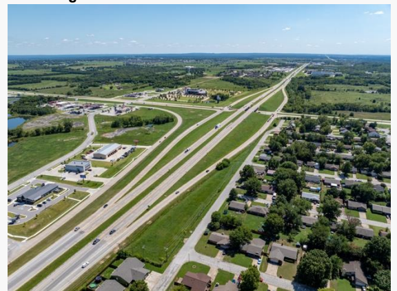
Looking Northwest at 151 st Street
