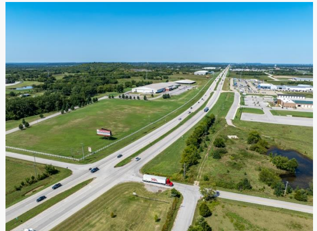
Existing US-75 Driveway Connections
