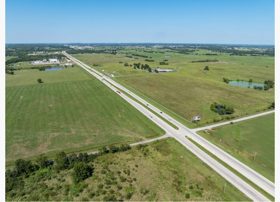
Looking Northeast at 191 st Street
