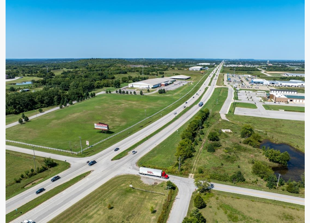
Existing US-75 Driveway Connections
